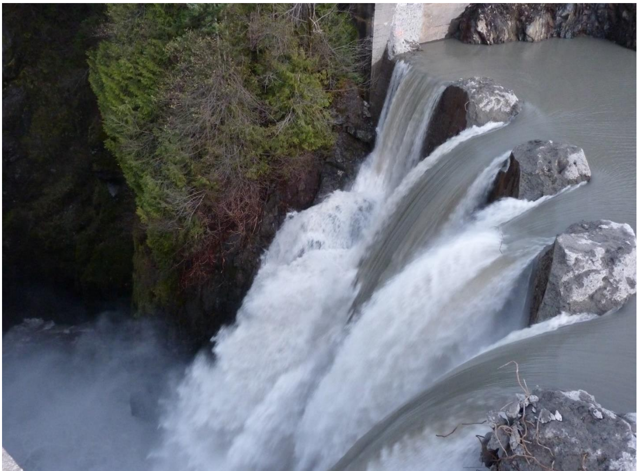
Glines Canyon dam removal, Elwha River (Washington State), 2014
